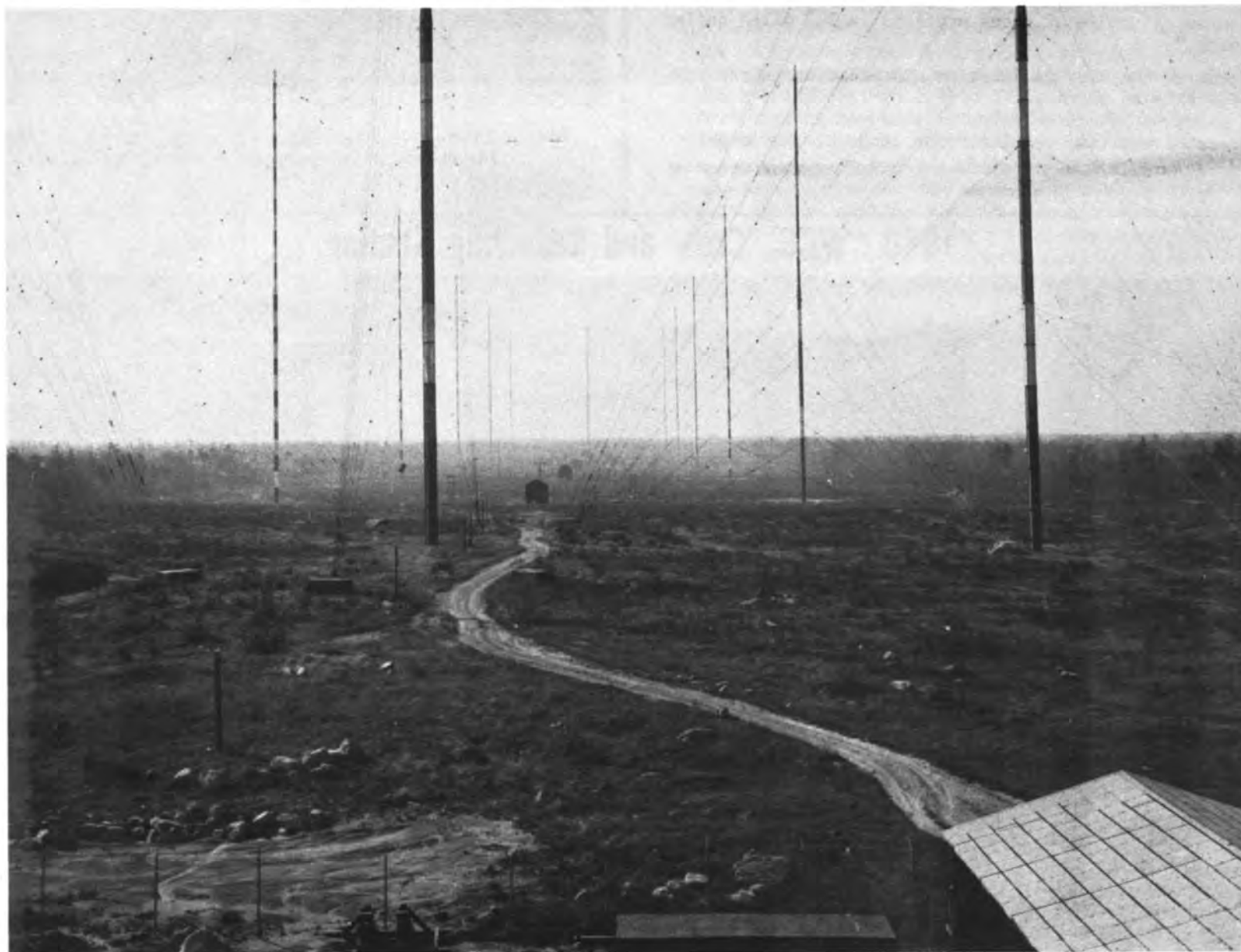
The Aerial system at Marion, Mass. These 300-foot tubular steel towers support a 24-wire horizontal directive antennass which are over 5,000 feet long. Tuning houses, similar to those at Tuckertwon, are located along the length of the aerial. This station was set up originally to transmit to Stavanger, Norway. The receiving station was located at Chatham, Mass. and received from Naerboe, Norway. An extensive radial ground system of copper wires is embedded in the ground under the aerial. Gaps in the ground wires have set fires in the peat-like earth in the past from excessive power used. On either side of each tuning house are frames that support a pulley and concrete counter weight arrangement for keeping wires to the tuning houses taunt. The system was set up by british Marconi in 1913, like the German scheme, was to be a part of a world-wide Wireless Empire. Pictures from the Lincoln A. Cundall collection furnished before his death.
